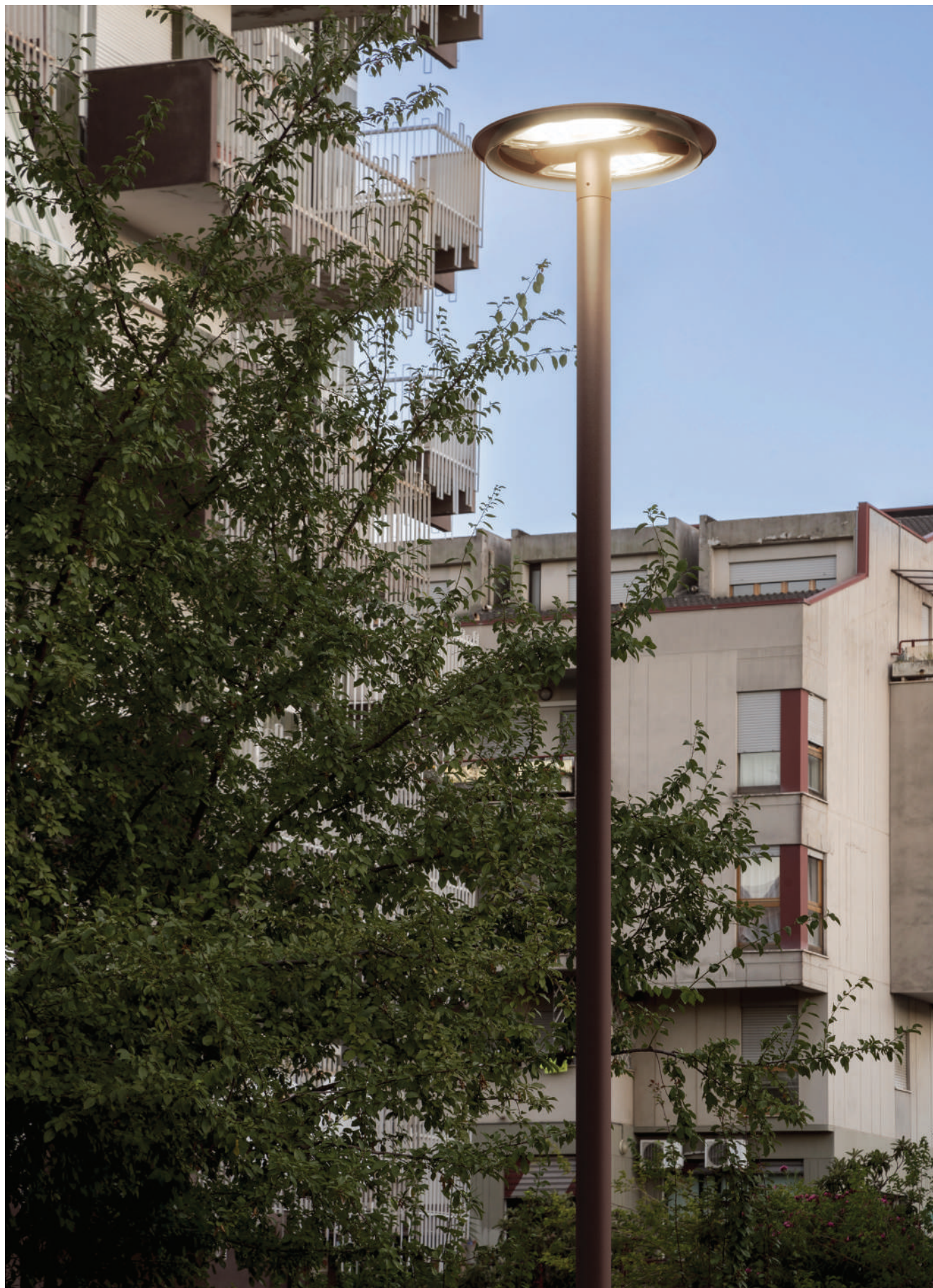
Public lighting relamping in Rende, Italy — Product: Twilight Calgary - Pole Top | Rust brown Ph: Stefano Ferrando, Studio Vetroblu
